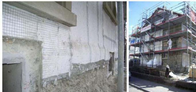
Another product developed by Aspen Aerogel is fiber composite cover, which is a flexible aerogel for thermal insulation. This product, which has low thermal conductivity, also has a fairly good load-bearing ability (Figure 17).
