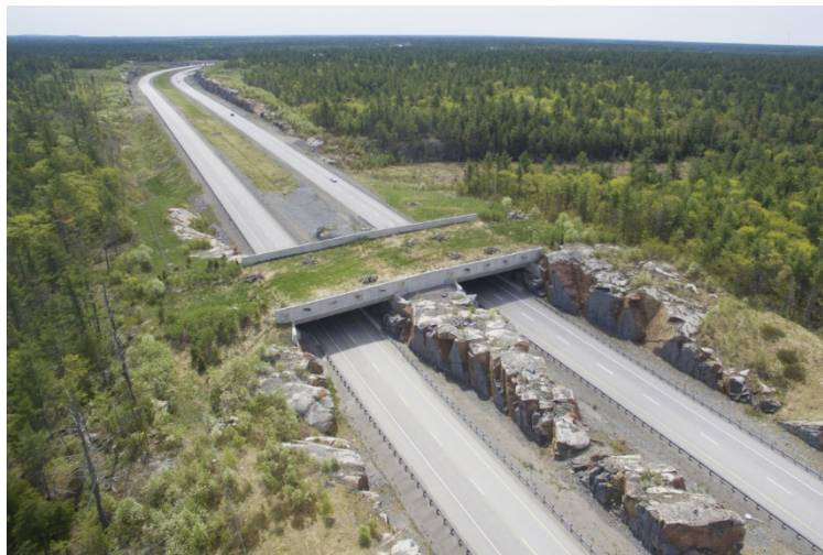
Figure 21. A Corridor Connecting Parts of the Habitat
