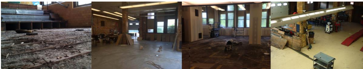
Figure 3. Learning environments prior to renovation and construction
